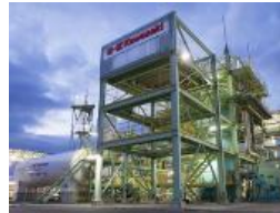
Hydrogen Liquefier Plant
