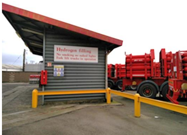
Figure 5 BOC Gases Ireland hydrogen production facility in Dublin
